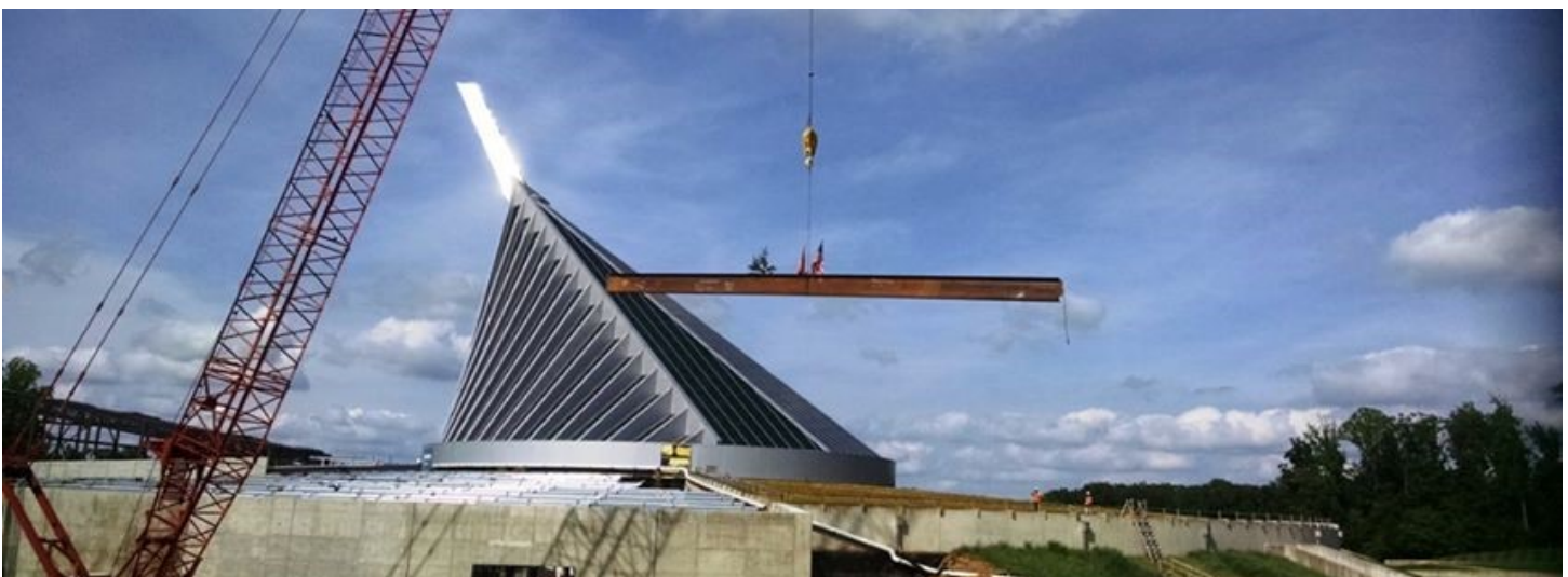
The final beam of the final phase is moved into place
