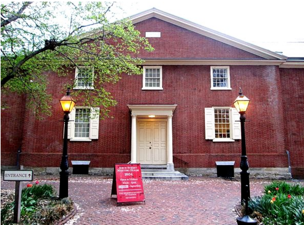
Arch Street Meeting House
