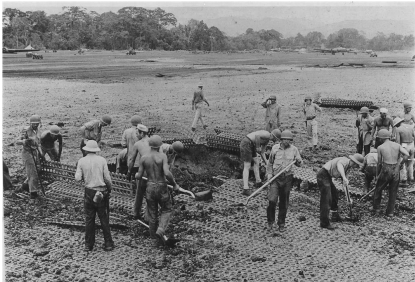
Henderson Field, Guadalcanal — Marston Mat damaged by Japanese bombs, 1942
